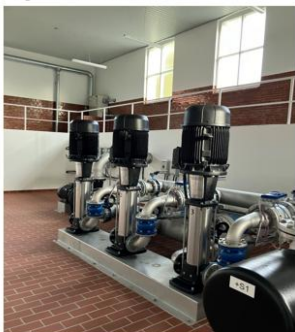
Figur 7 – Rentvandspumper
