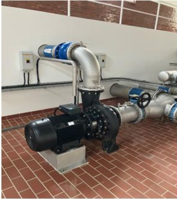
Figur 9 – Skyllvandspumpe
