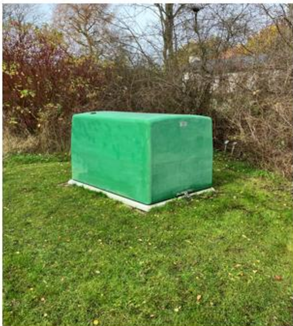
Figur 13 – Overbygning Boring DGUnr. 194.992
